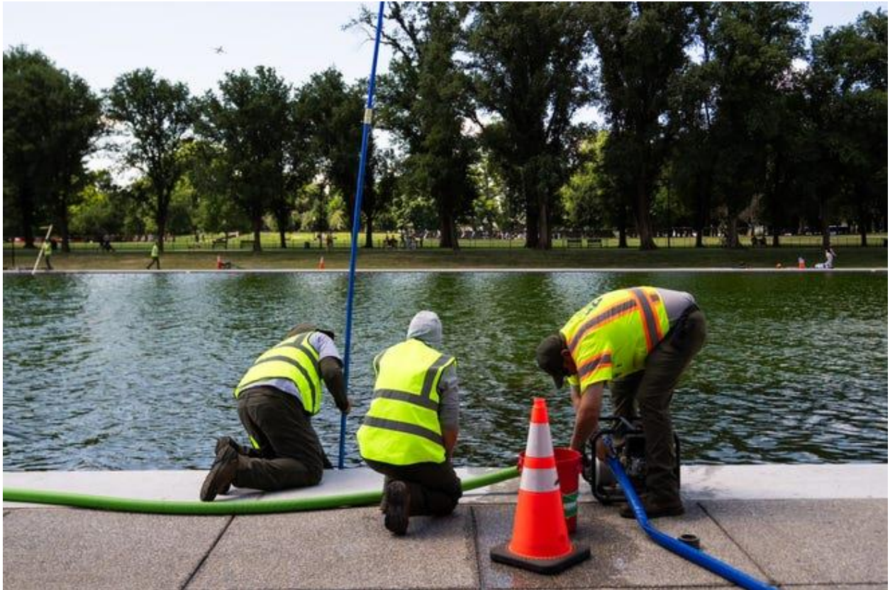
Crews use nanobubbler treatment and vacuuming to clear algae from the Lincoln Memorial Reflecting Pool, which turned green shortly after a June renovation.
